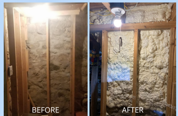
RIGHT: basement walls in old farmhouse before (uninsulated) and after (insulated).
